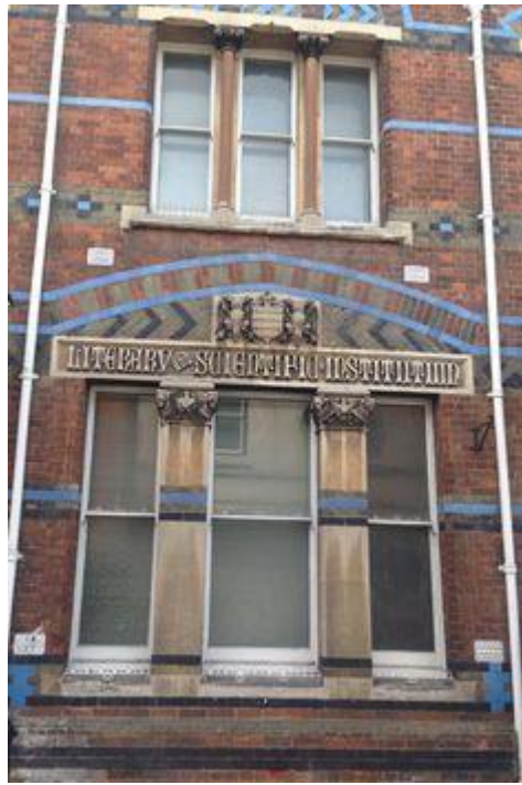
Typical Institution Building
