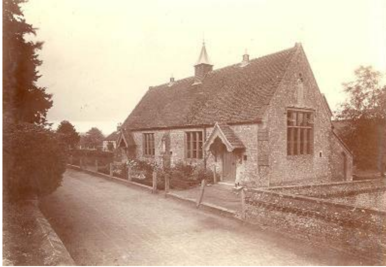
The National School at Longbridge Deverill, c. 1905
